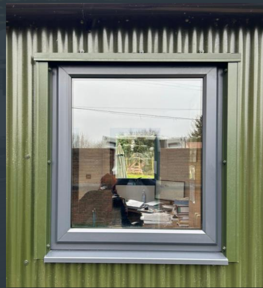
Fire Wall Cladding
